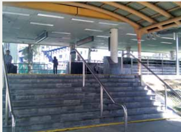
Minimum crest levels are required for entrances to underground facilities such as Mass Rapid Transit (MRT) stations.
