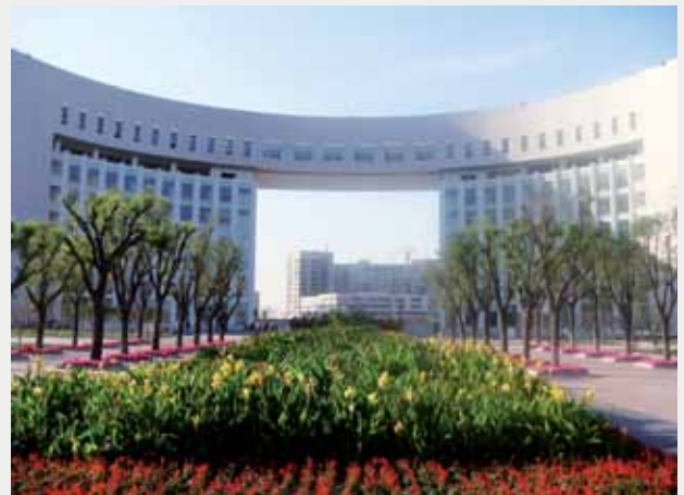
In pursuing sustainable growth, Singapore has built capabilities that are relevant to other cities facing similar sustainability challenges. The National Animation Park in Tianjin Eco-city is an example.
