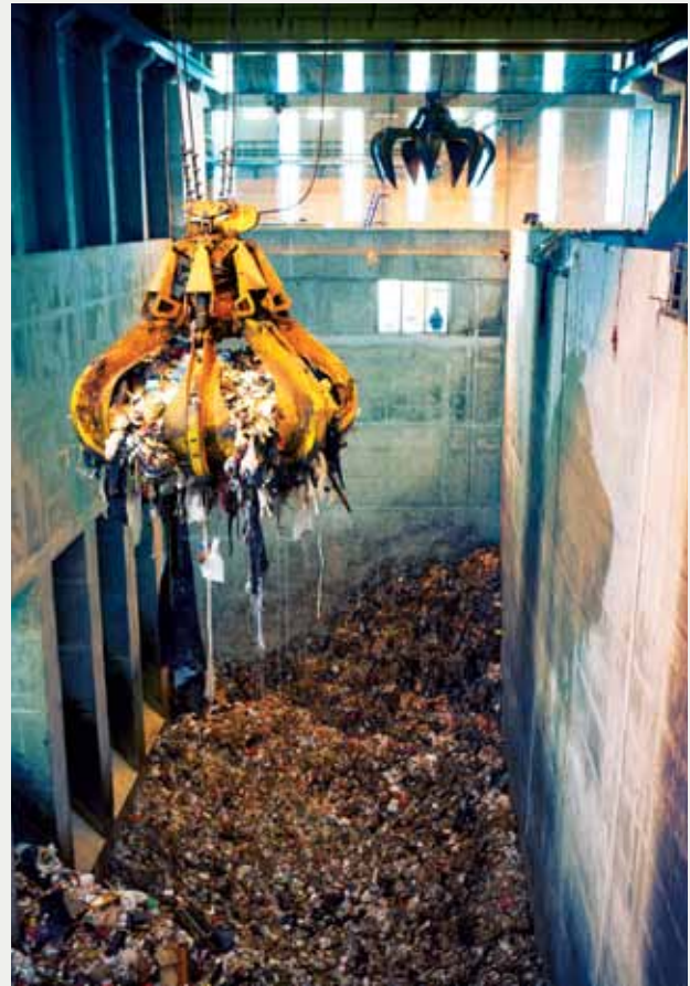
Waste being prepared for incineration at the Keppel Seghers Tuas Waste-to-Energy plant. Besides diverting waste from landfills, incinerating waste also recovers heat energy that is used to produce and supply electricity to homes and factories.
