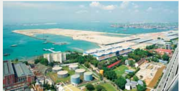
Minimum platform levels for new reclamation projects were increased to cope with potential rising sea levels.
