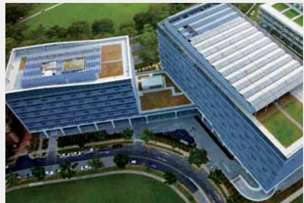
7 & 9 Tampines Grande, a commercial development, incorporates the use of Building Integrated Photovoltaic (BIPV) Panels (dark-coloured) on the building façade, as well as Photovoltaic Panels (dark-coloured) and Solar Thermal Panels (light-coloured) on the rooftops.
