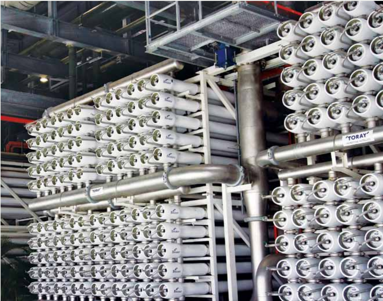
Reverse osmosis membrane systems are used in the production of NEWater, an ultra-clean and high grade of reclaimed water. It will form an important component of Singapore's future water supply.
