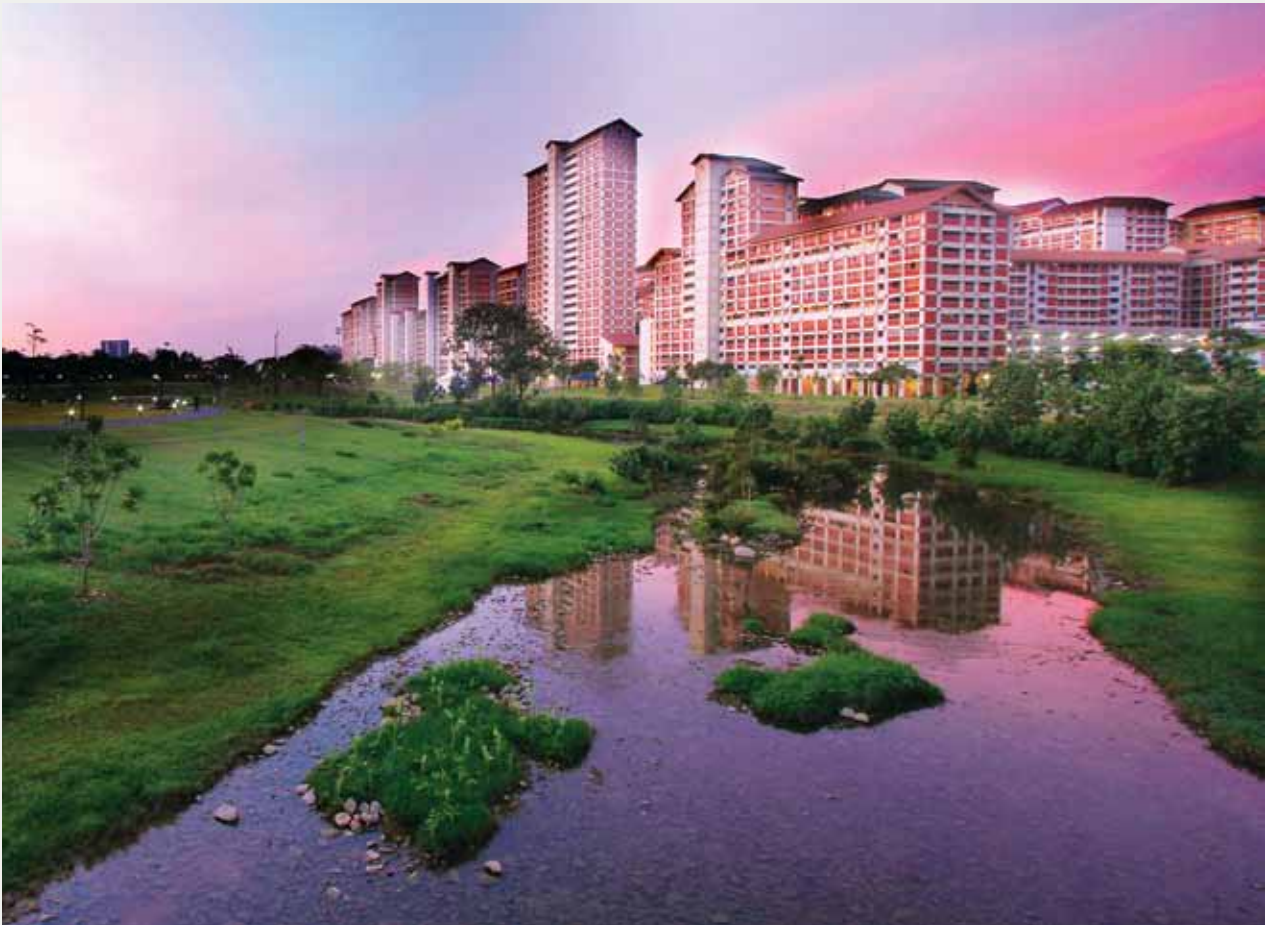
Naturalised river meandering through the newly-revamped Bishan-Ang Mo Kio Park—a project undertaken by PUB under the Active, Beautiful and Clean Waters (ABC Waters) Programme.
