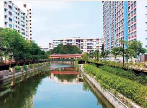
Continual drainage improvement works, which include expansion of drains and canals, are carried out to ensure the adequacy of Singapore's drainage system.
