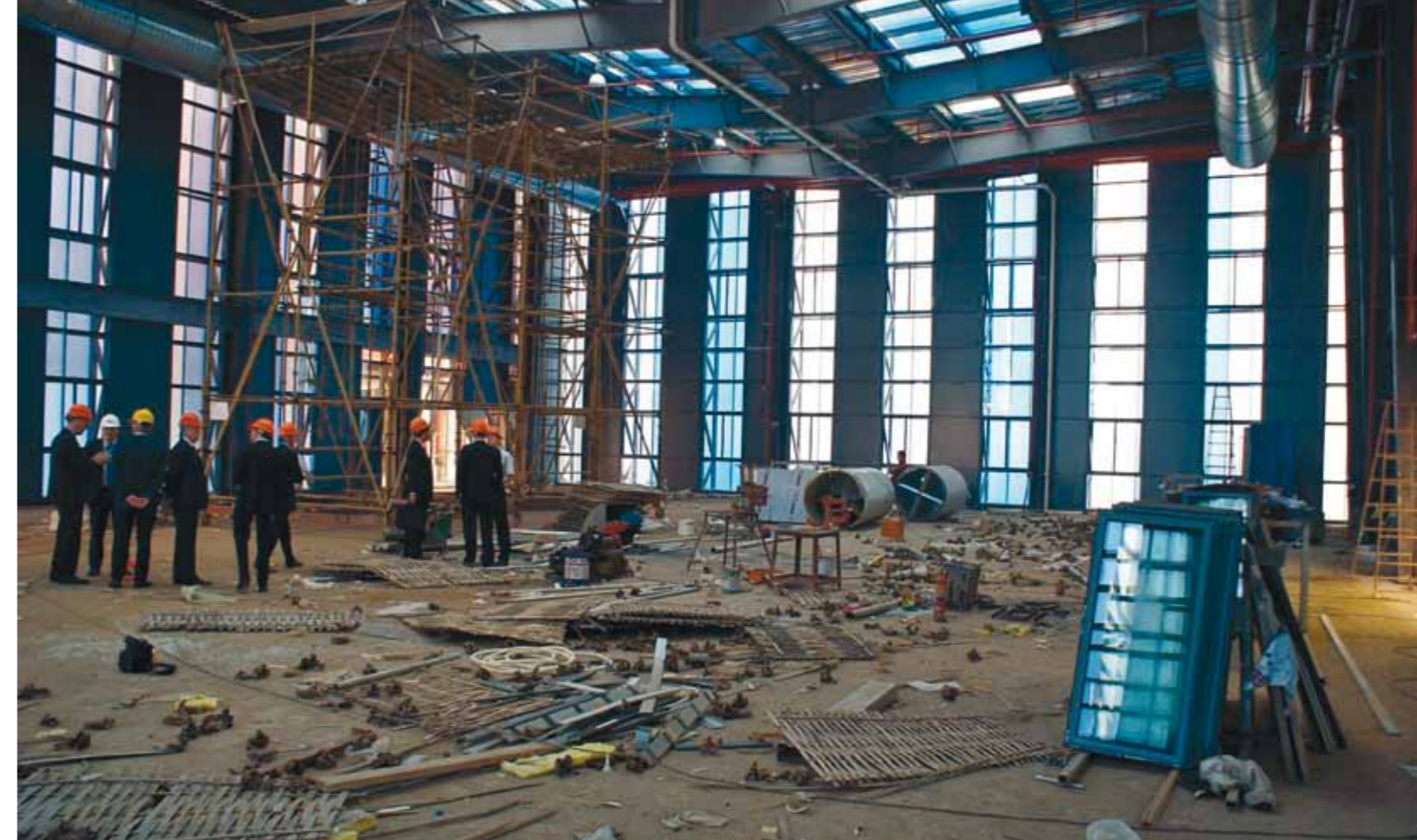
Construction of the 'Rotterdam Water City' pavilion, World Expo Shanghai 2010
